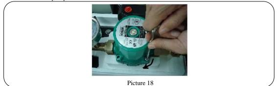
• Connect the power supply again and close the terminal box.
